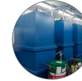
Tanks for bulk liquids that are pumped out to hose reels, and the transport of waste liquids.
