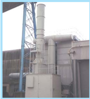
Cutting, trimming and finishing gypsum products
