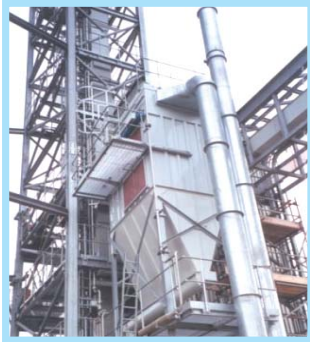
Dockside handling, conveying and storage, of grain
