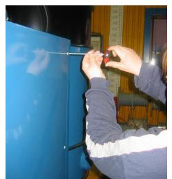
30) Refit the rear panel. NOTE! Refit the lower corner screw.
