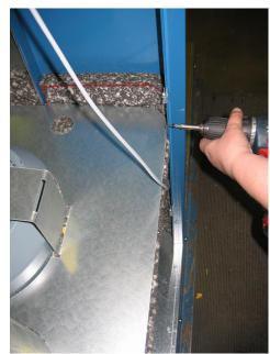
15) Unscrew the three remaining sheet metal screws securing the blower cover and remove it so it does not interfere with the blower (tilt up and out).
